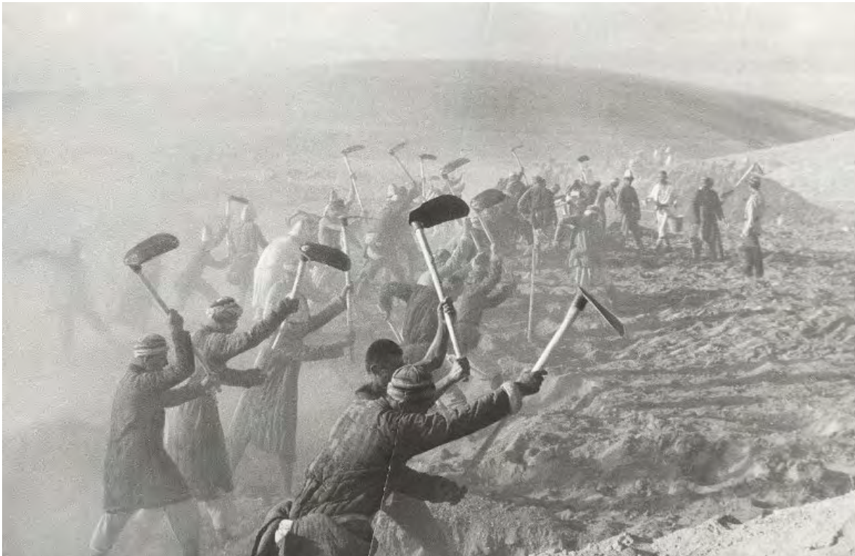
Construction of the Great Fergana Canal. Source: Max Vladimirovich Alpert, 1939.
