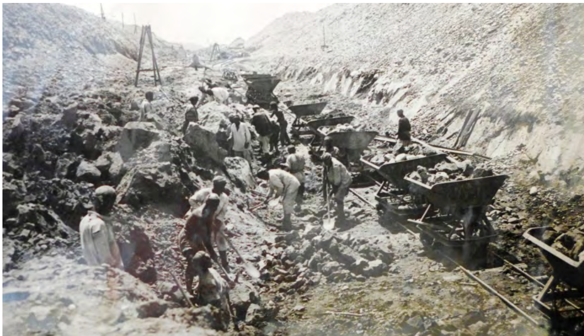
Volunteers from all over the Union of the Soviet Socialist Republic (USSR) participated in constructing the Vakhsh principal canal, an offshoot of the Vakhsh River.
