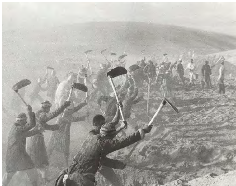
Construction of the Great Fergana Canal. Source: Max Vladimirovich Alpert, 1939.
